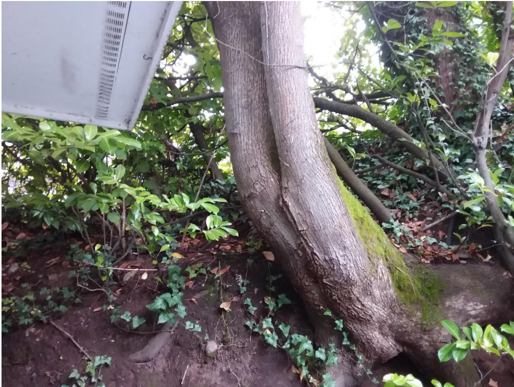
Figure 4. Base of #1 maple showing the separation point and proximity to the SW corner of the existing garage.
